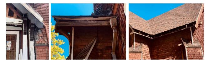
Stage 1: Repair Roof Leaks, Stop Wood Rot, and Address Eave Damage
